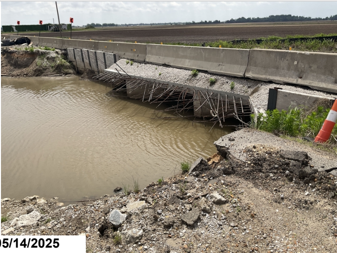
North end of culvert, stage 1 construction.
